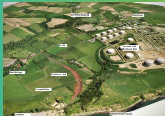
Waterston and Blackbridge Highways
